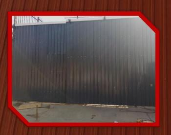
Lastly we have a gate and fence that we cladded due to the inferior sheets that were used before as well as damage that occurred.
