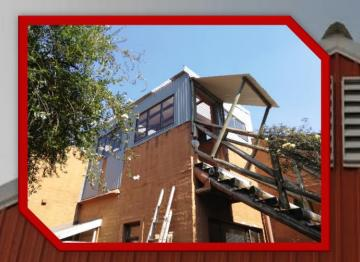
The middle picture was a 2<sup>nd</sup> story balcony that we turned into an office with cladding and sheeting to fit in with the rustic staircase.
